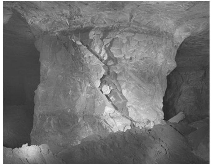
Figure 10. Partially benched pillar that failed along two prominent discontinuities dipping at approximately 60°.
