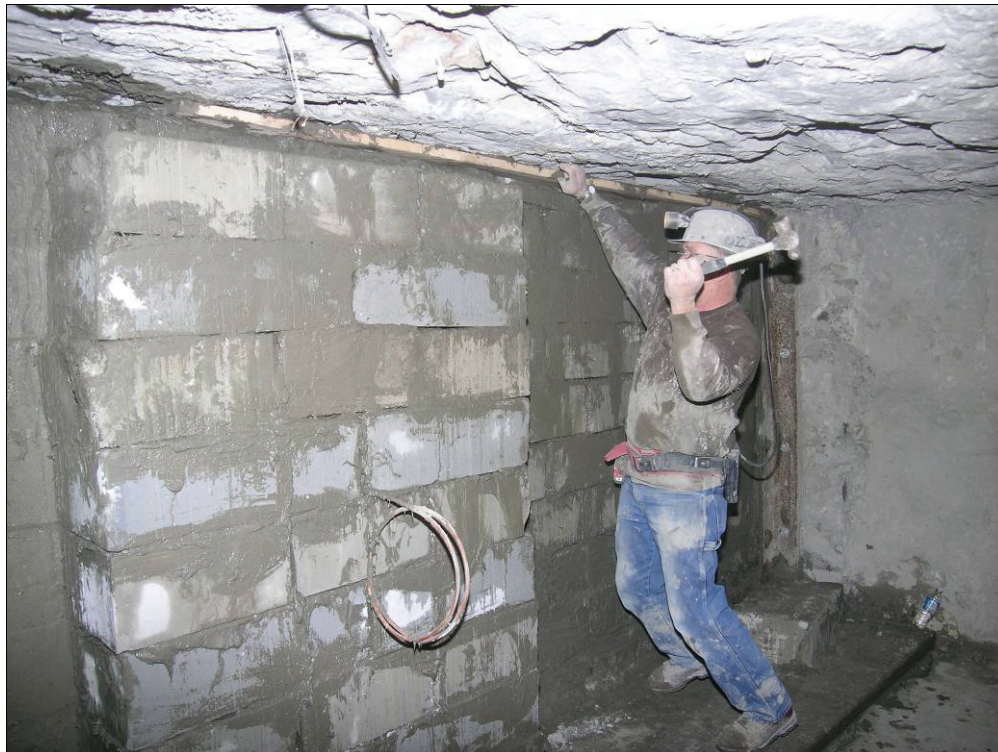
Figure 15.—Installing the wood planking on the top course of block.
