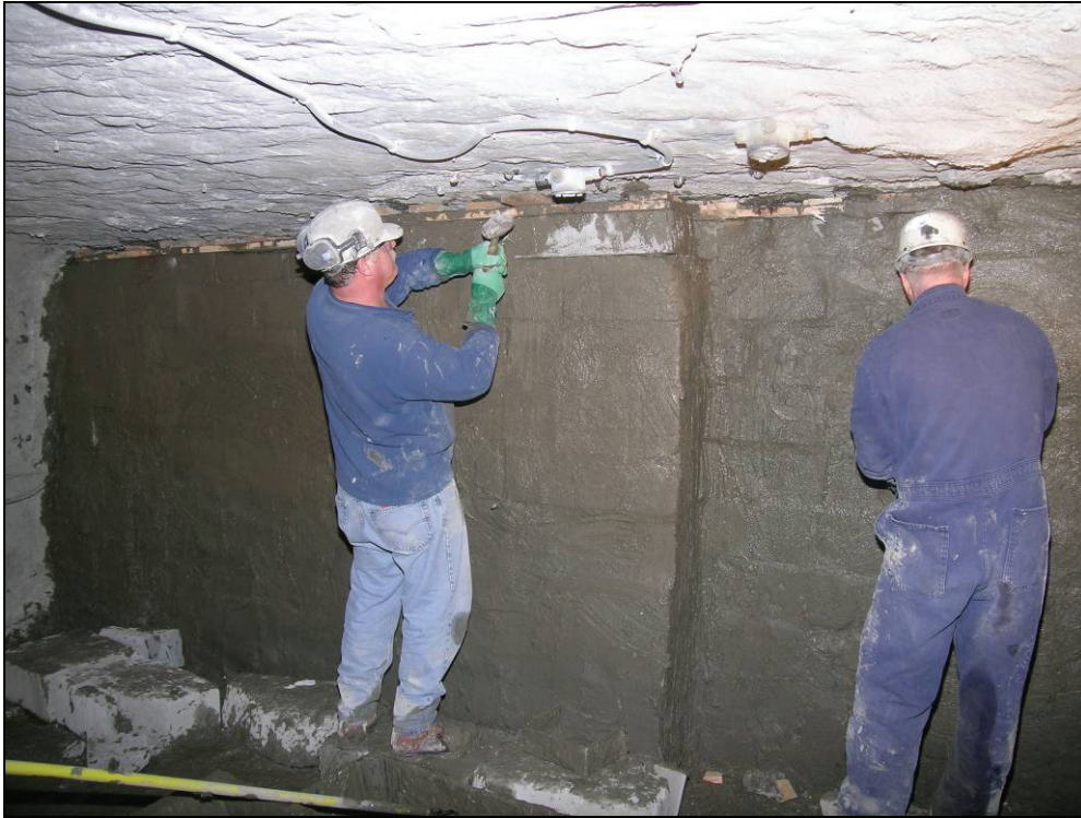
Figure 16.—Wood wedges driven perpendicular between the mine roof and wood planking.
