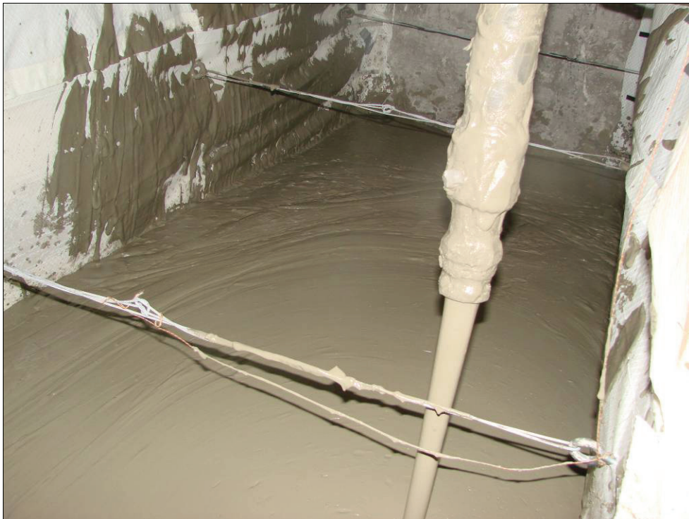
Figure 9.—Pumping of cementitious foam slurry between form walls.
