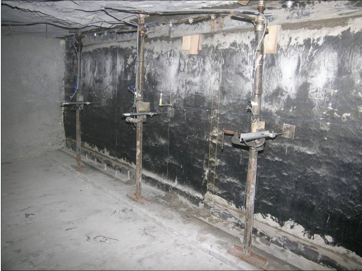
Figure 28.—Completed CFRP reinforcement retrofit to the crosscut 3 low-density block seal.
