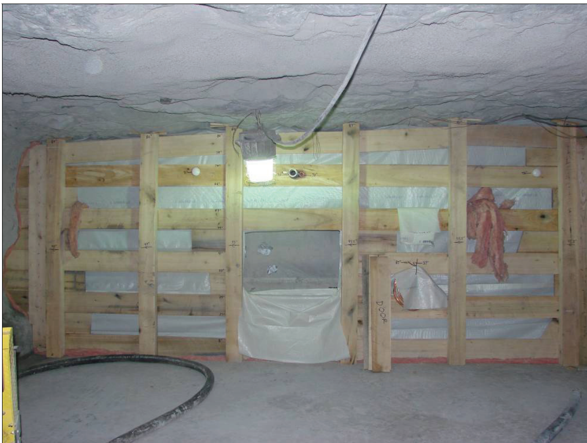
Figure 6.—Outby form wall for the pumpable cementitious foam seal.
