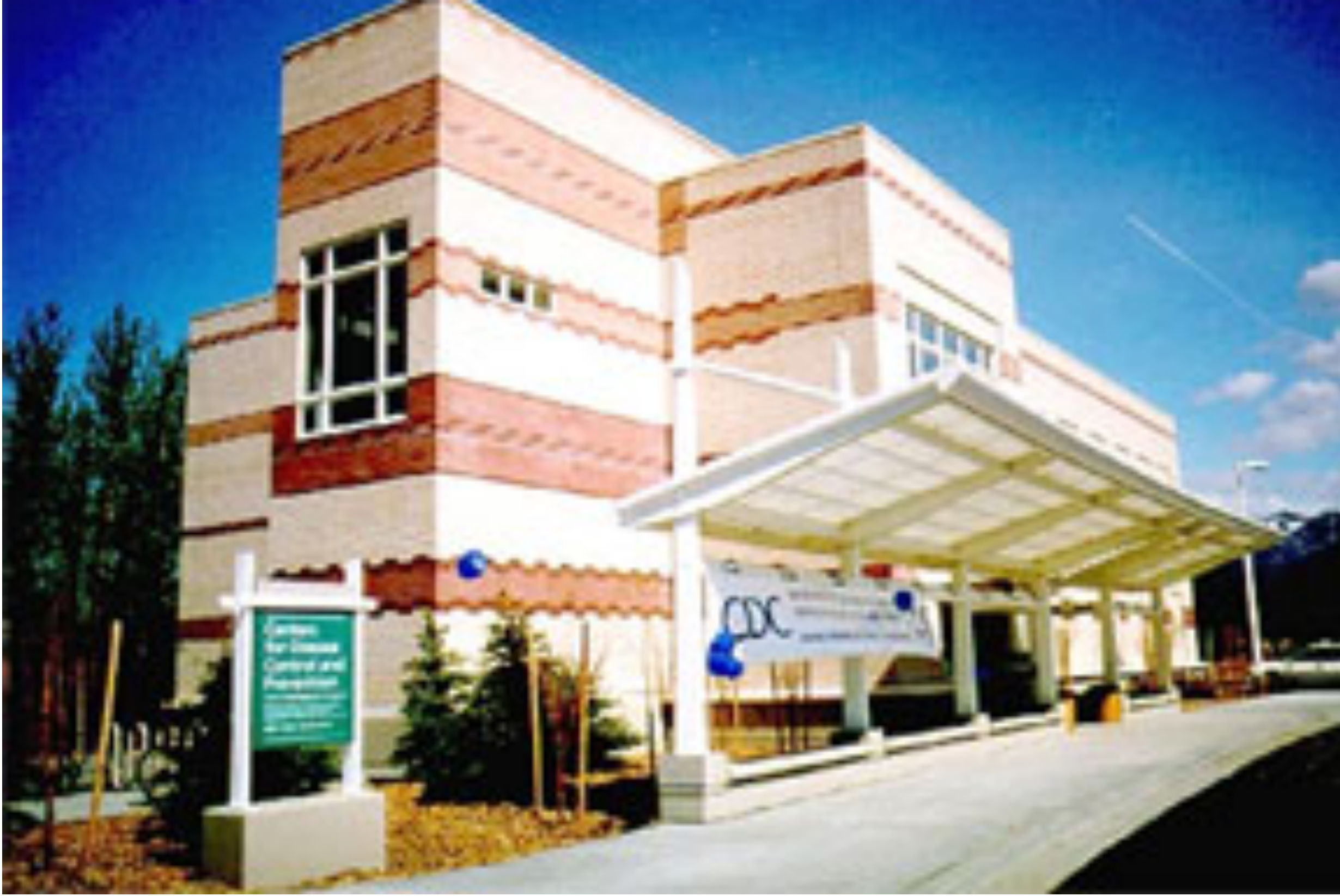
Current AIP building.
