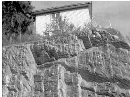
Figure 18.—Examples of rock masses with particularly low CC (left) and particularly low FC (right). These require relatively more shotcrete (left) and relatively more bolting (right). The original Q-system case records have apparently reflected these different needs, and the Q-parameter ratings developed have given the possibility of realistic CC and FC values.
