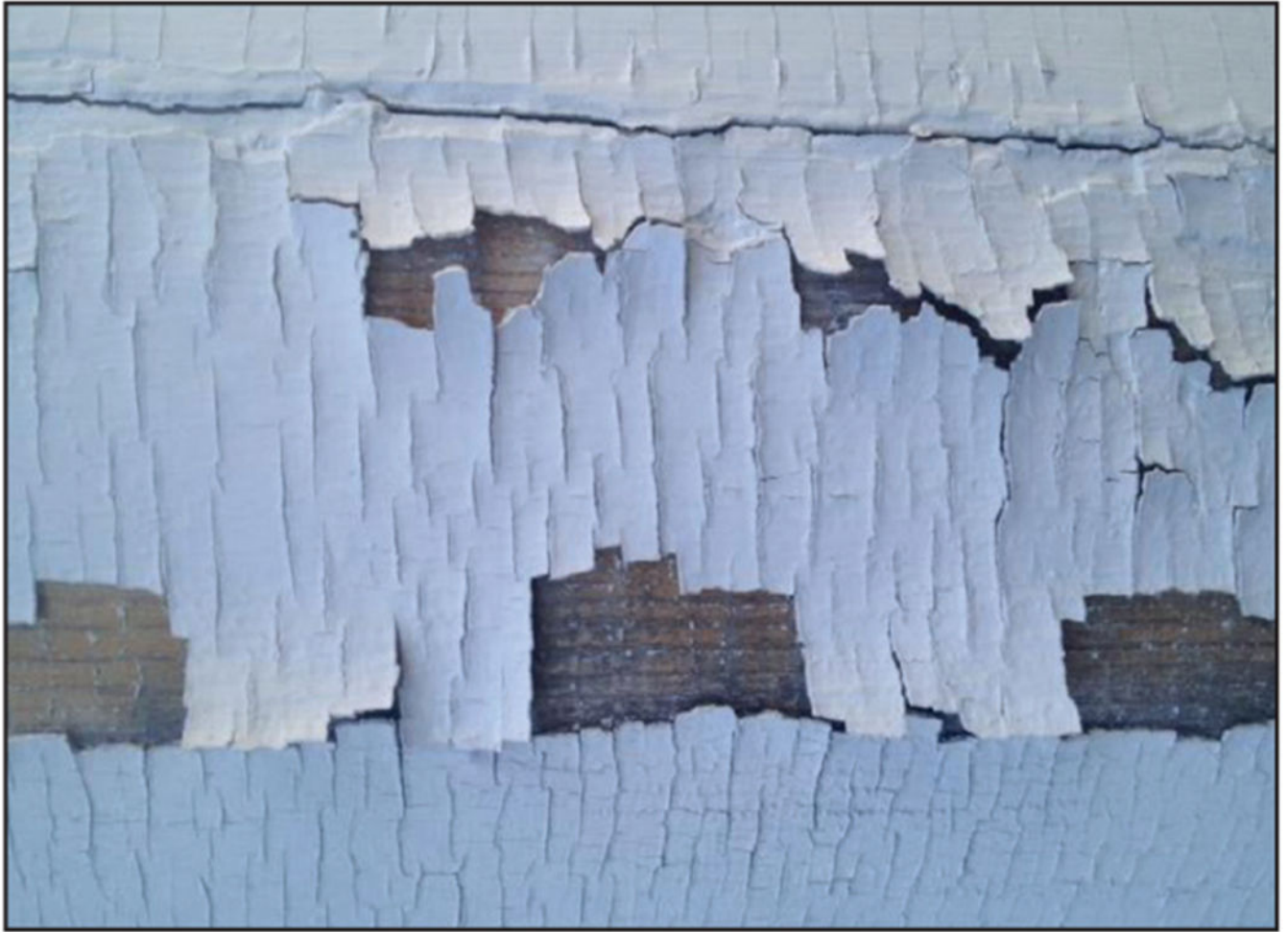
Figure 1. Example of peeling lead paint. The toxic chips can be ingested by infants and toddlers.
