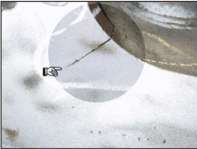
Figure 14.—Failure of base rib side plate where fabrication process left large flaws.
