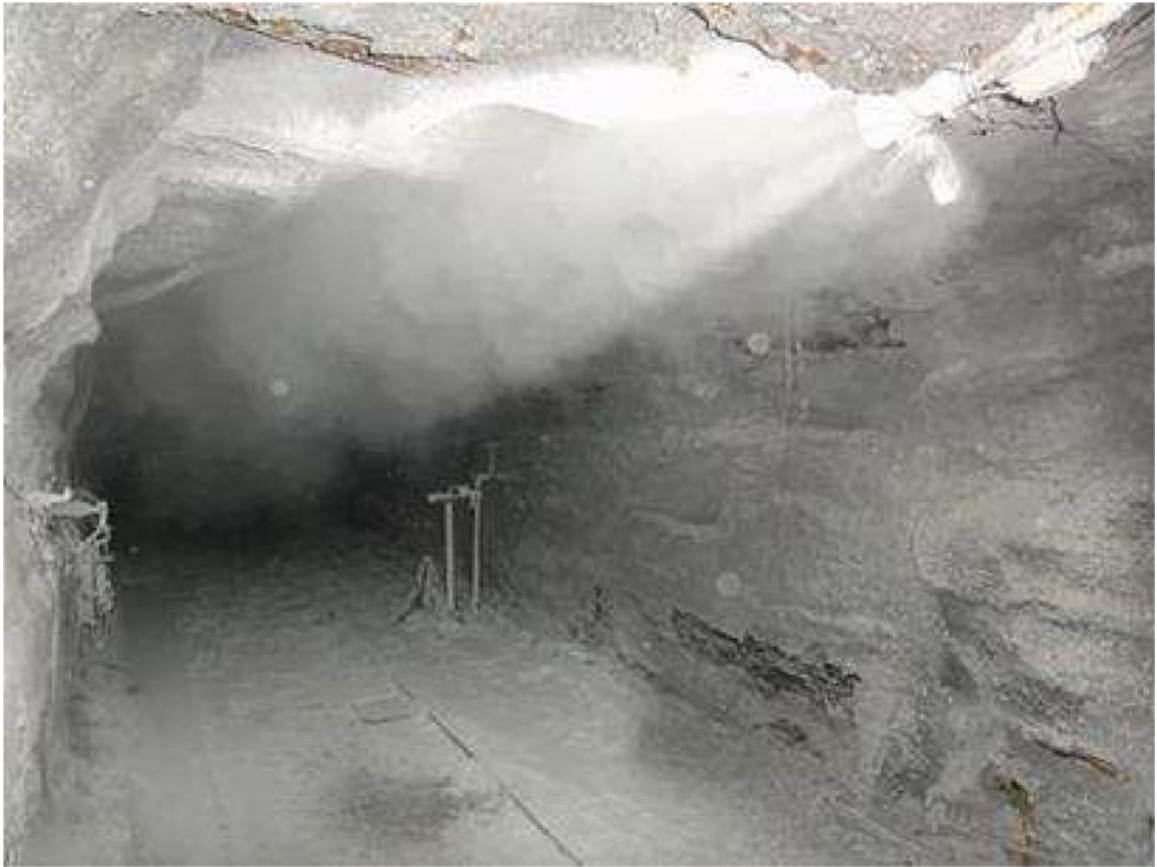
Figure 2. Air-dust discharge through a 2-in (5.1-cm) diameter tube attached to the roof 7.25 ft (2.2 m) above the floor
