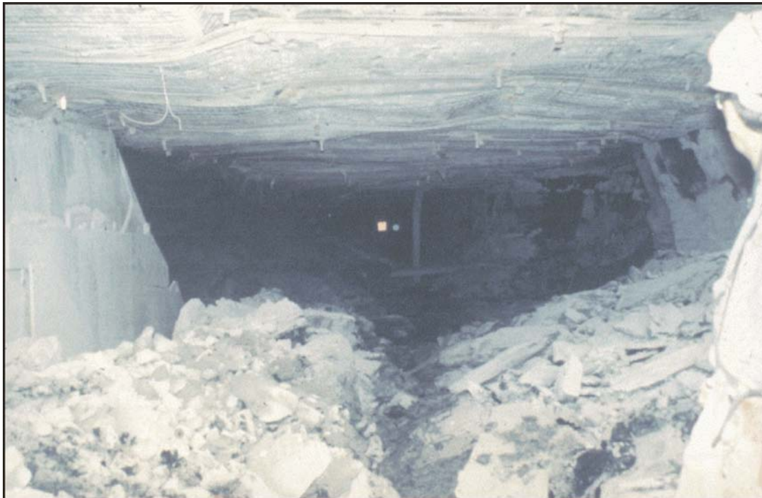
Figure 17.—Tailgate behind the shields kept open with cable bolts.
