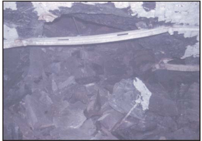
Figure 16.—Tailgate behind the shields has caved though supported with cable bolts.
