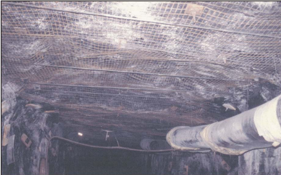
Figure 26.—Cable trusses installed in the headgate entry.
