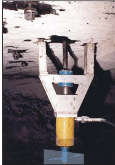
Figure 4.—A smooth hole lowers anchorage strength, as seen with this bolt as it pulls out of the hole.
