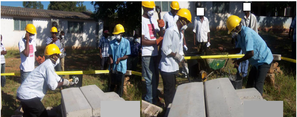
Figure 5. Photo of workers (one mason and two assistant masons) sprinkling water before breaking up concrete/masonry structure and pushing a wheelbarrow filled and covered with plastic sheet (after the training to use checklist) (Photographer: C.M.).
