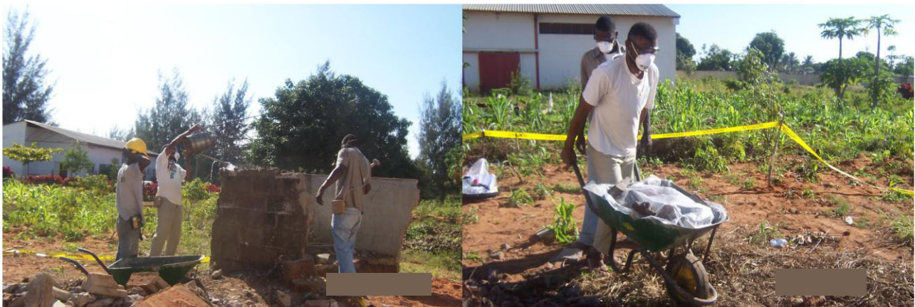
Figure 5. Photo of workers (one mason and two assistant masons) sprinkling water before breaking up concrete/masonry structure and pushing a wheelbarrow filled and covered with plastic sheet (after the training to use checklist) (Photographer: C.M.).
