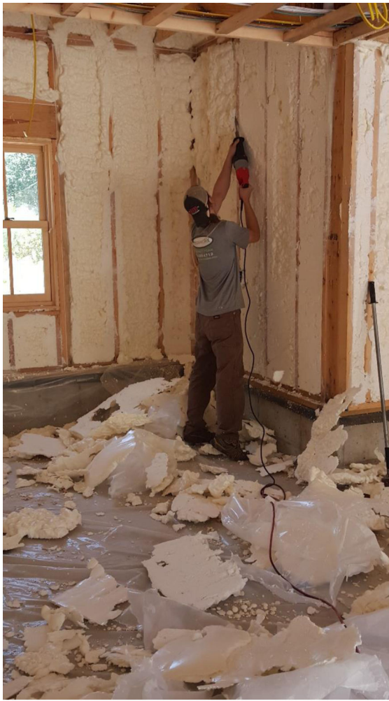
Figure 1. Photos of helper (left) and sprayer (right). The helpers cut and bundled freshly sprayed foam, sometimes without coveralls or gloves. The sprayer usually wore partial coverall, gloves, and an air-supplied respirator for protection from overspray.
