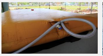
Figure 7.5-4. Onion water tank with removable cover
