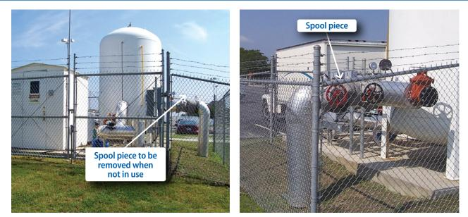
For accessible explanation of these two images about spool piece to be removed when not in use, and location of spool piece see Appendix G.
