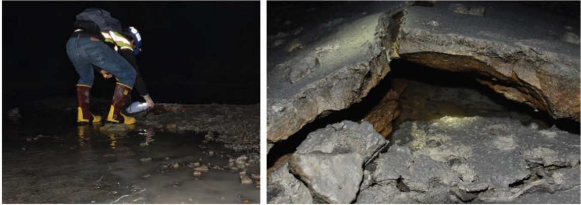
Figure 3 - Floor buckling.
