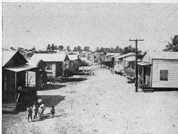
Ratproofing by elevation in Puerto de Tierra.
