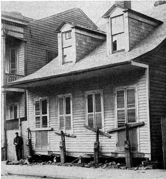
Ratproofing by elevation of buildings, New Orleans.
