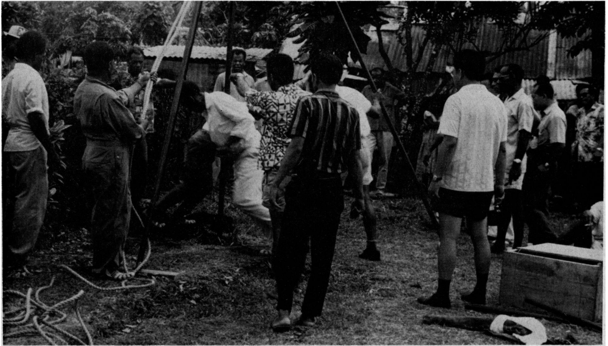
Class exercise in constructing bored-hole latrine
