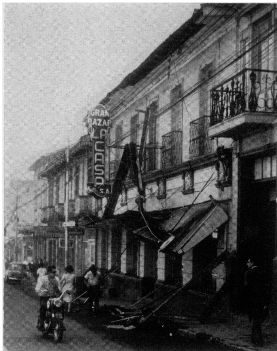
Figure 3. Collapse of roofs and roof gutters caused by ashfall from eruptions of Irazú Volcano, San José, Costa Rica, December 1963
