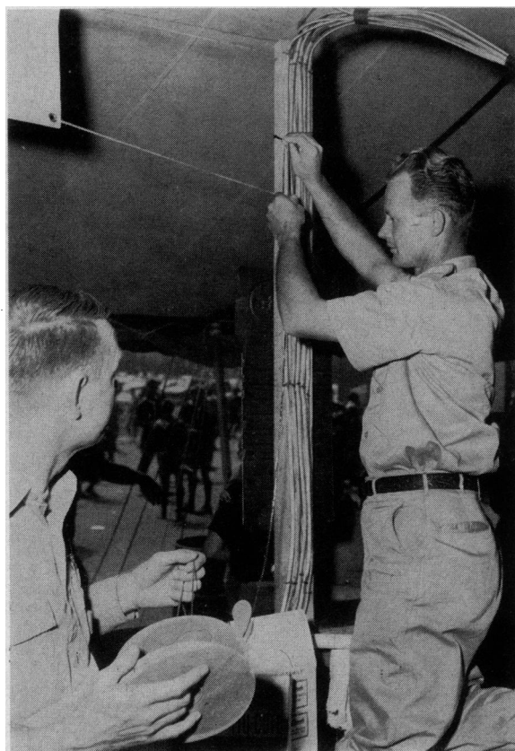
Insecticide-impregnated cord is installed in a food serving area. A staple tacker is used to attach the cord to counter struts and posts.
