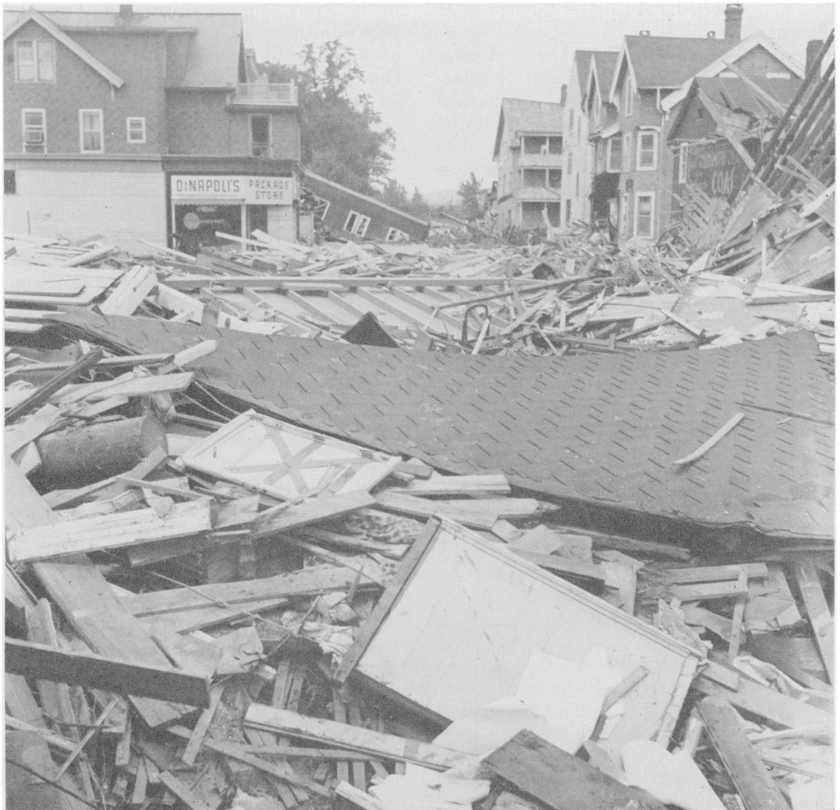
Shattered, splintered avalanches of debris settled on city streets as flood waters roared through Waterbury, Conn. Food stores and other sources of necessities became inaccessible islands in a sea of wreckage like this.
