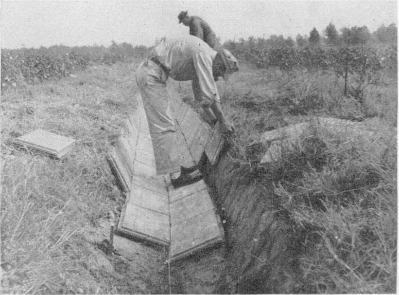
FIGURE 16.—Laying a 3-slab-wide V-bottom ditch lining in a previously shaped ditch.
