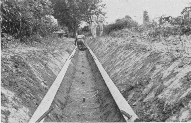
FIGURE 3.—Ditch prepared for lining. Note forms and center-line stakes in place.
