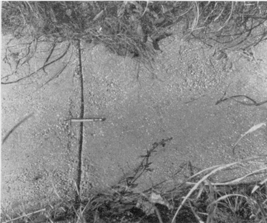
FIGURE 8.—Dummy or false transverse joint.
