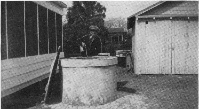
FIGURE 2.—A "10-day" inspector spraying a cistern with kerosene.
