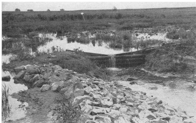
FIGURE 5.—Small earth-filled dam constructed to produce Harris Station experimental pool, Wheeler Reservoir.
