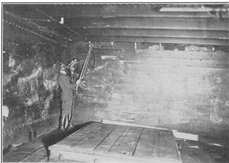
FIGURE 6.—Projecting HCN spray directly into rat-infested insulation of a cold-storage room. The apparatus shown is the first one used, in which the handle and valve were assembled separately. A strip of casing has been removed to permit direct application of fumigant to insulated space
