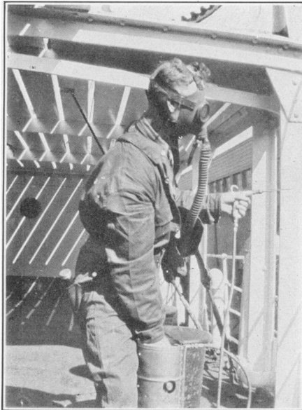
FIGURE 4.—Dosing cylinder with hand air pump and measuring device for dosing small compartments
