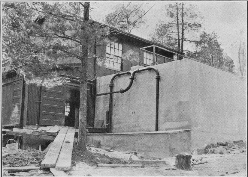
Fig. 3.—Air supply pipes to channels under filter plates
