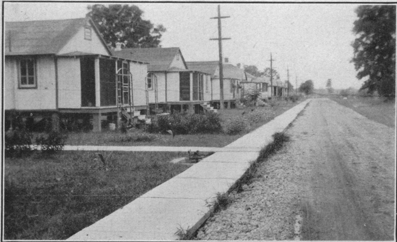
Concrete walks, serving also as covers for the conduits carrying the steam and water pipes
