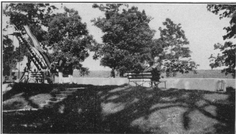
Outdoor swimming pool, constructed by officers and attendants
