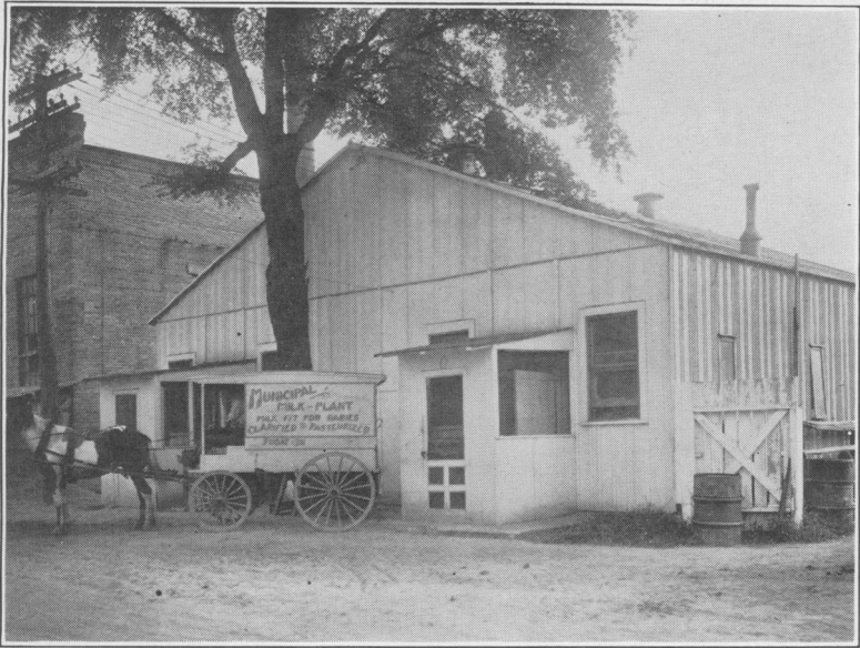
Municipal Pasteurizing plant, Tarboro, N. C.
