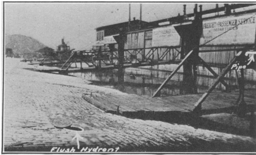
Levee at Memphis, Tenn., showing a flush hydrant, with cover removed, near the end of the landing stage, ready to be connected by hose to the pipe on the landing stage leading across wharf boat to steamer
