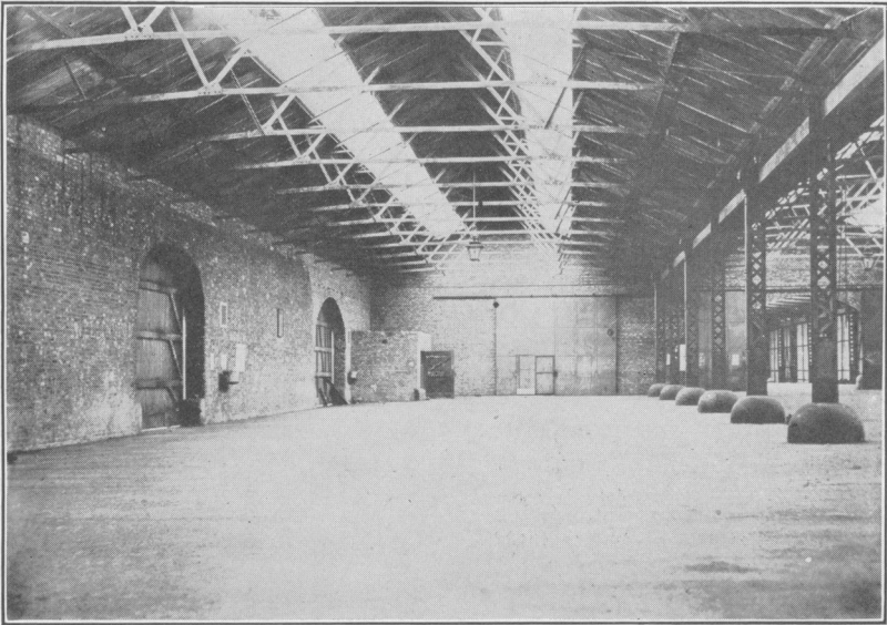
Rat-proof storehouse on dock estate at Liverpool, England
