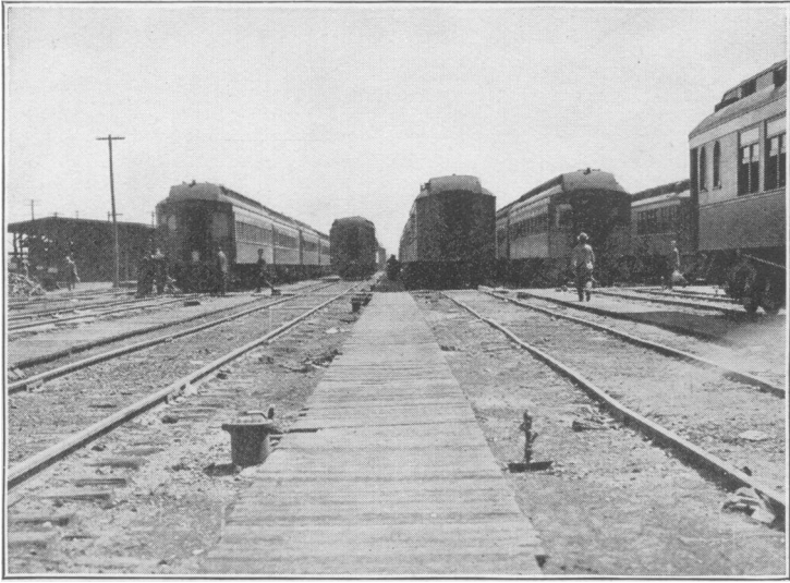
A. Section of "through" coach yard with plank walks. When steam lines are laid under these wooden walks, rats nest under them in winter. Note that hydrants are so located that pollution by toilet wastes from cars is possible.
