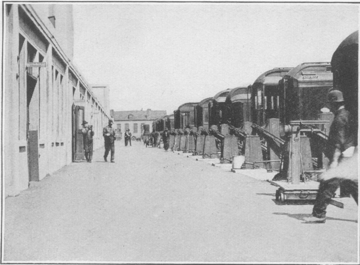
B. End walk of "terminal" coach yard. Steam and hot and cold water are available at track terminals. This is an exceptionally clean coach yard.
