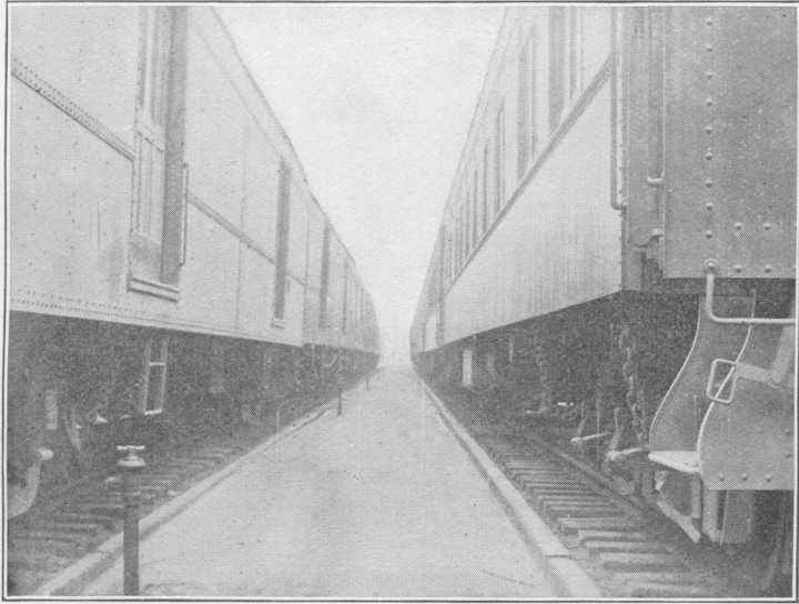
A. Brick walk between tracks in coach yard, with concrete gutters for draining water used in washing cars. Note location, spacing, and height of hydrants.
