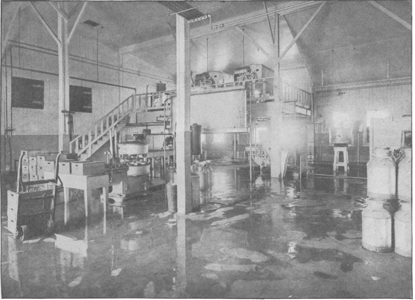
Fig. 4.—Manufacturing and bottling room, Reconstructed Milk Plant, Nitro, W. Va.
