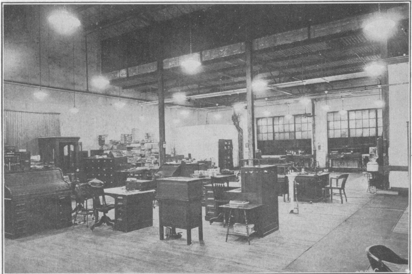
Fig. 14.—A factory office illuminated by a general system of lighting, arranged to conceal brilliant light sources. Adequate light is provided without drop lamps at the desks. (See also Fig. 15.)
