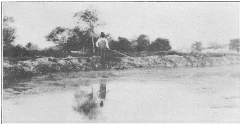
FIG. 9.—TREATING POND WITH COPPER SULPHATE FOR KILLING ALGÆ. LABORER IS DRAGGING A SMALL BAG OF THE CHEMICAL THROUGH THE WATER BY MEANS OF A POLE.
