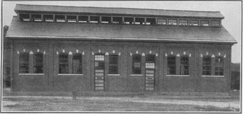
A. CHANGE AND WASH HOUSE AT EDGEWATER, ALA
