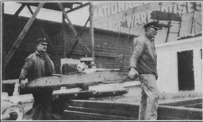
CARRYING THE FAN. THIS MAY BE DONE WITH MACHINE RUNNING.
