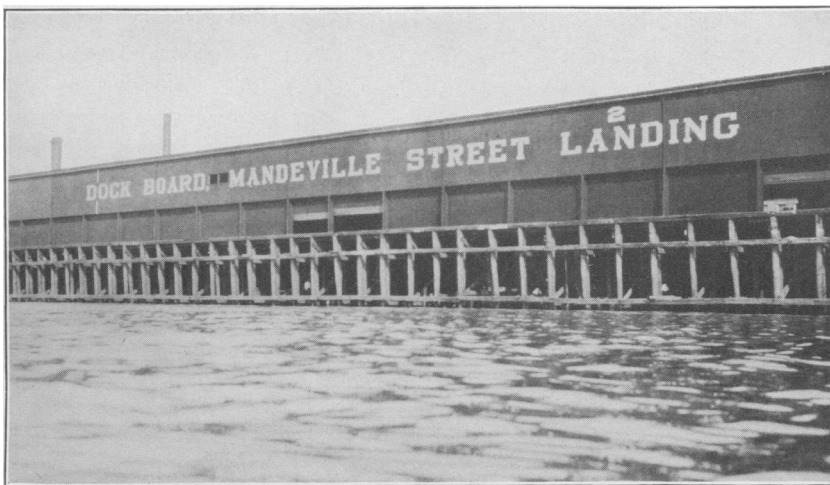
FIG. 1.—TYPICAL WHARF AND SHED AS SEEN FROM RIVER.
