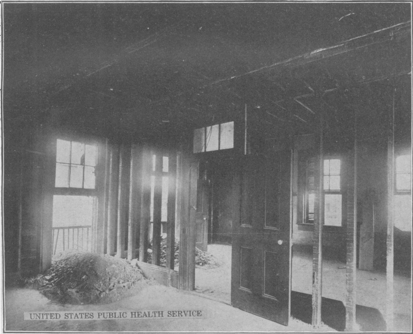
FIG. 5.—SHOWING DEMOLITION ON SECOND FLOOR OVER RESIDENTIAL PORTION.
