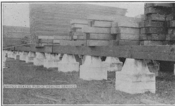
FIG. 2.—RAT-PROOFING LUMBER BY ELEVATION ON CONCRETE PILLARS
