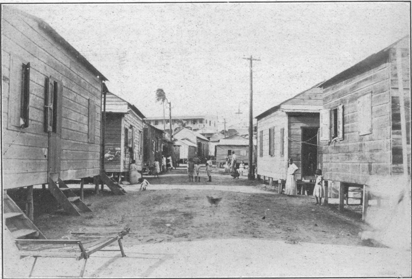
Fig. 9.—SCENE IN SOUTH PUERTA DE TIERRA SUBSEQUENT TO RAT PROOFING BY ELEVATION.
