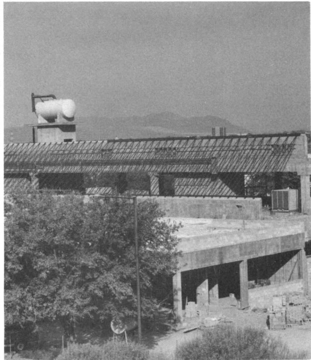
Framework for solar collectors on new health facility
