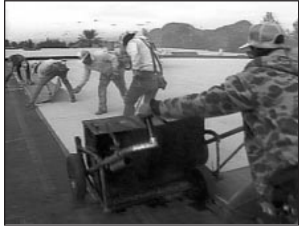
Figure 3–6. Mechanical felt-laying machine
