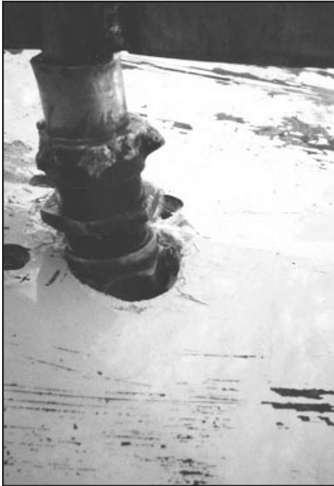
Photo 1: A Failed Rudder Post Housing
