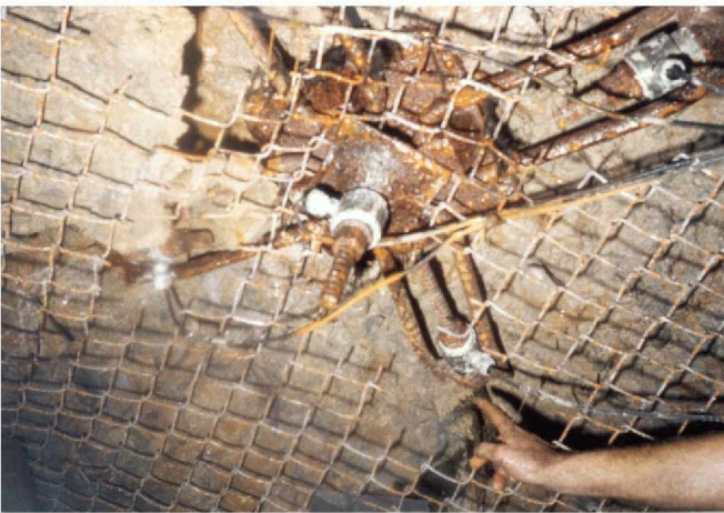
Figure 17.—Load cells at truss four-way bracket.
