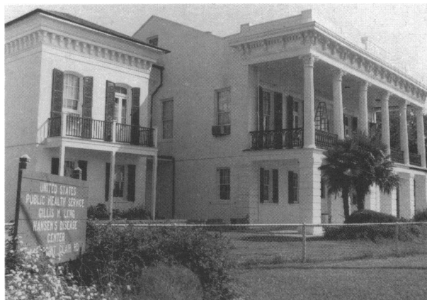
The original Indian Camp Plantation home (1857) now serves to house the office of the Director and other functions of the Gillis W. Long National Hansen's Disease Center. (courtesy, Hansen's Disease Center)
