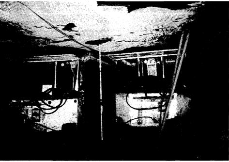
Figure 1.—Mobile roof supports in operation.
