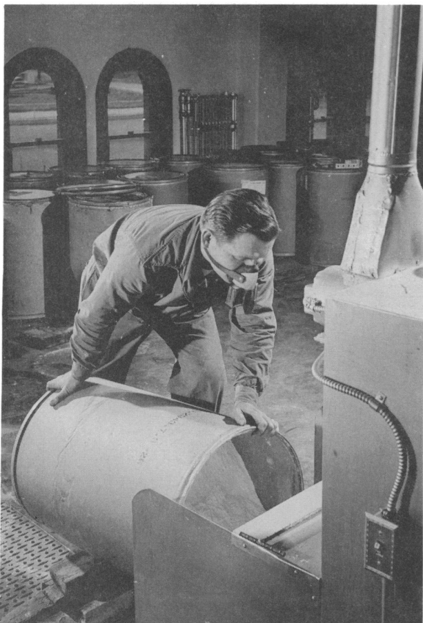
A worker adds fluoride to water in Grand Rapids, MI, in 1945 as part of the first community water supply experiment to demonstrate the efficacy of the caries prevention treatment
