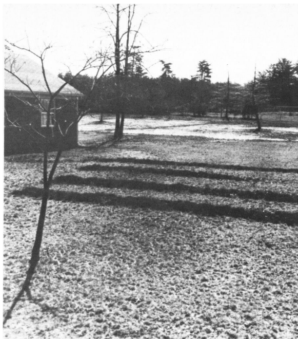
Darker colored grass outlines the septic tank drainline of a system beginning to fail
