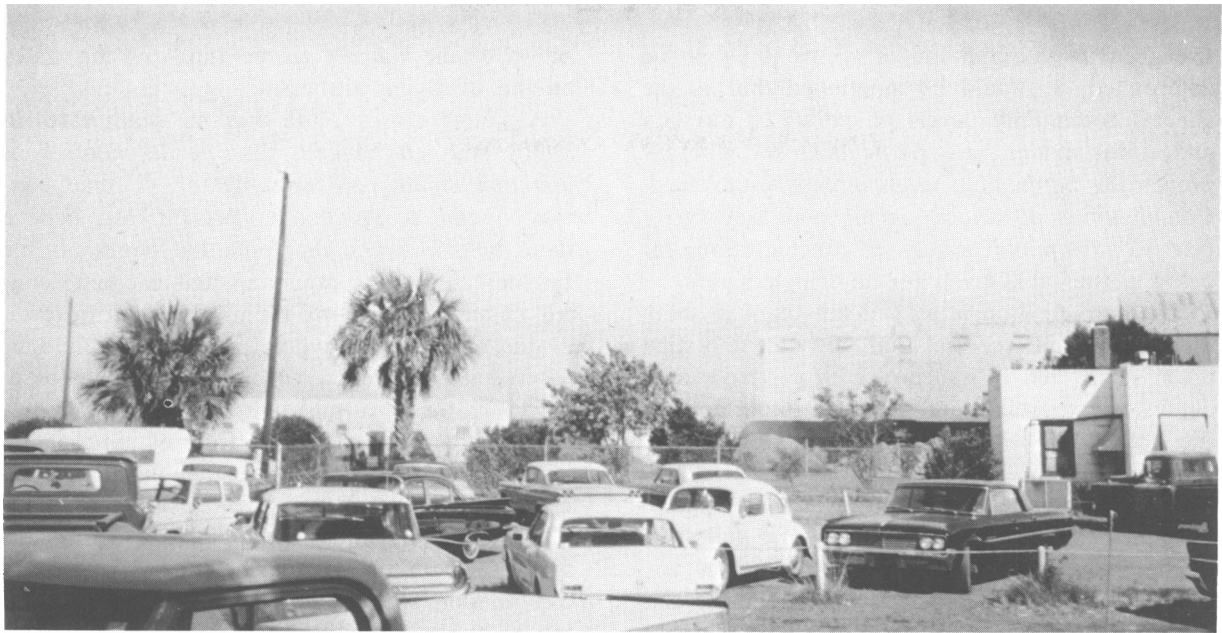
In 1968, emissions from ferroalloy plant completely obscured background on Charleston Peninsula. Below, March 1972, same area as above after new $17 million plant had been built
