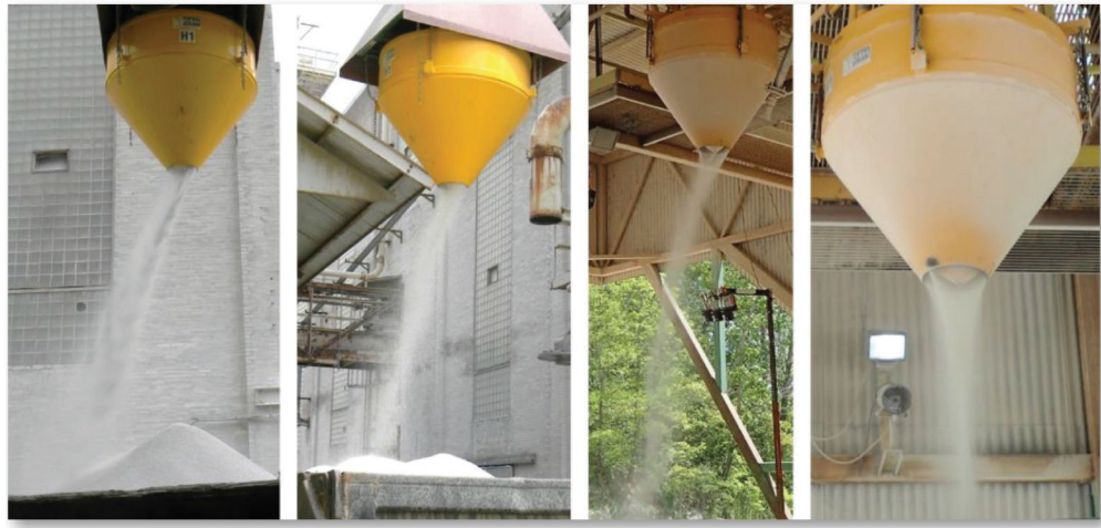
Figure 8. Silica sand discharging from DSH as loading ends.
