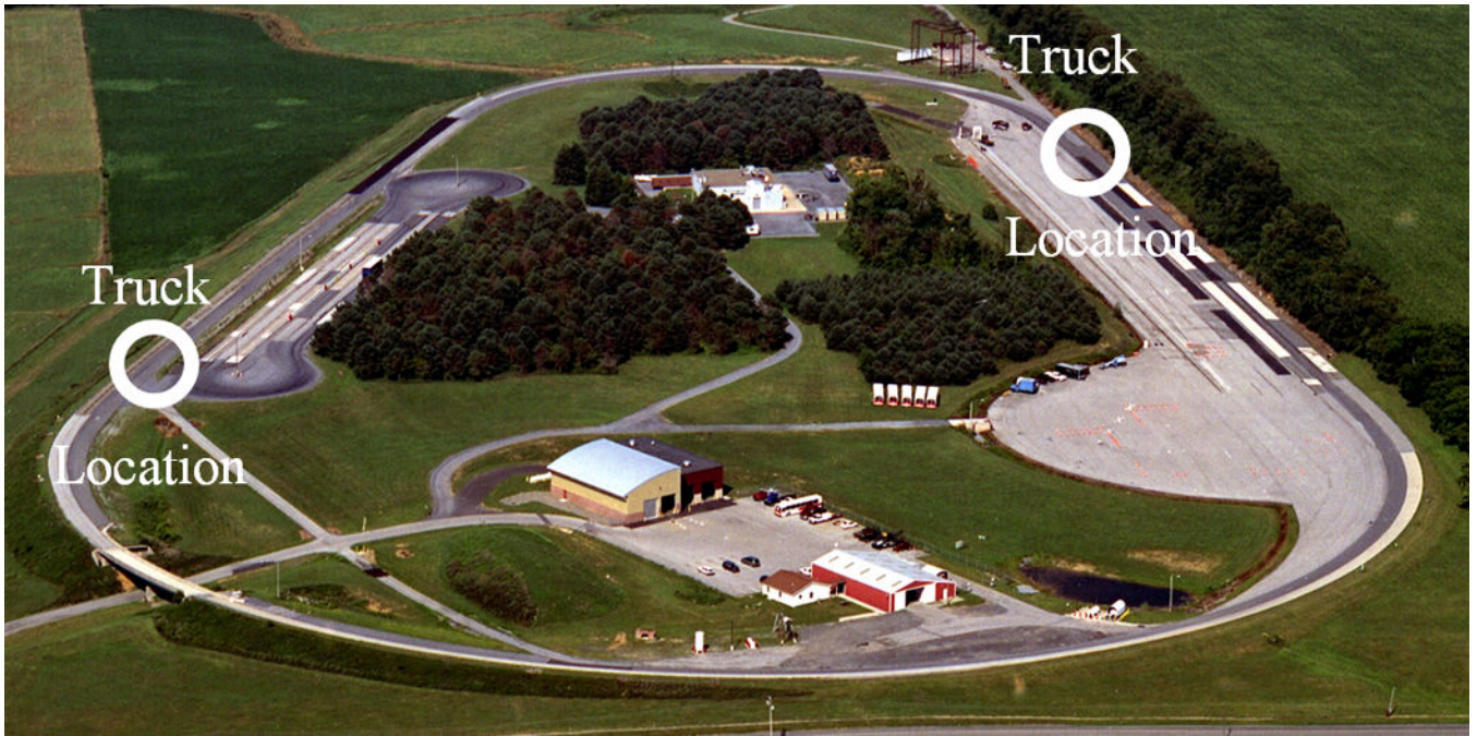
Figure 1. Penn State's Thomas D. Larson Pennsylvania Transportation Institute Test Track.
